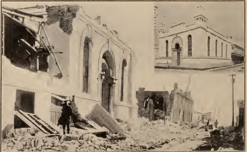
THE PRESBYTERIAN CHURCH BEFORE AND AFTER
